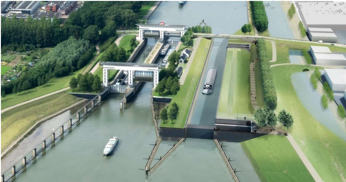
ASSET MANAGEMENT TERNEUZEN LOCK
